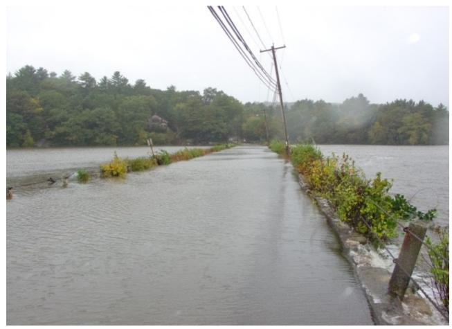
The image above shows the causeway looking west on the evening of October 14, 2005; in the lower corner on the right you can see the water rushing down the north side of the causeway. By morning of October 15, part of the causeway was washed away. \2/ The concrete post in the lower right corner is shown in another picture below from a different angle in a picture taken today, on March 6, 2022.
