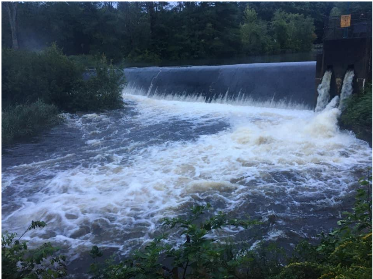
Hamilton Reservoir Dam- September 2, 2021- Photo Credit: Holland Police Department Archives
