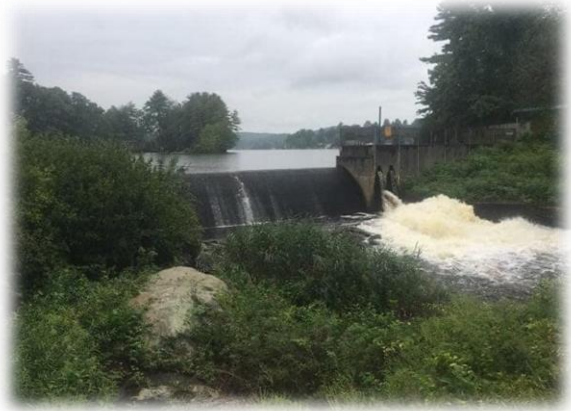
Hamilton Reservoir Dam- September 2, 2021 Photo Credit: Holland Police Department Archives
